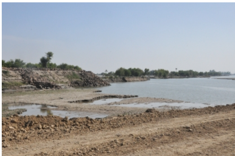
View from the Ring Bund of the un-pitched portion of the breached embankment at Taunsa (05---10---2010)
